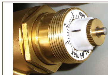
Dial under actuator used to set limit to maximum flow
