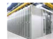
Shanghai Dingyi datacentre
